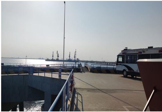
拟建码头西侧 (已建滚装船码头)
